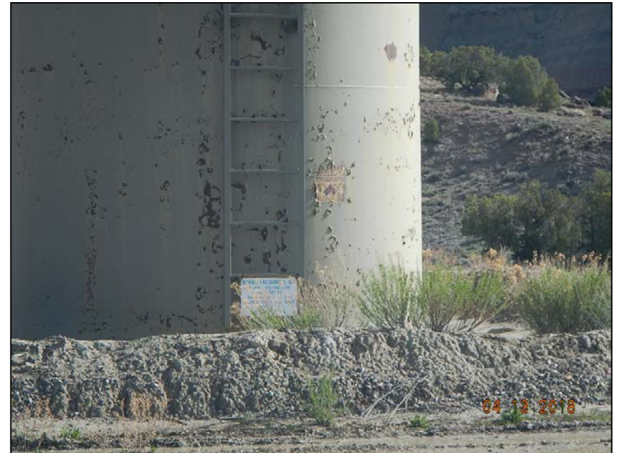
Photo 2. Vegetation in containment and tank sign not legible.
