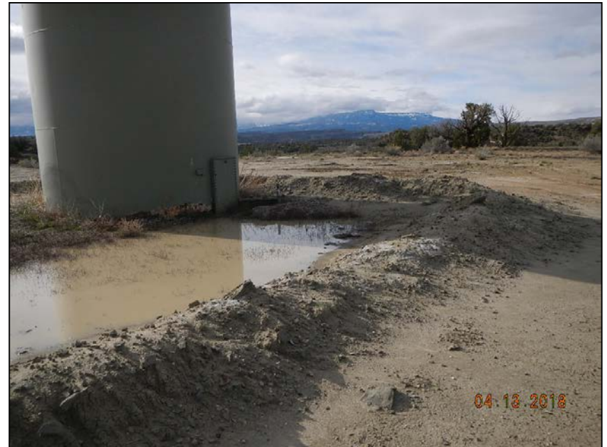
Photo 2. Eroded/washed out area of berm.
