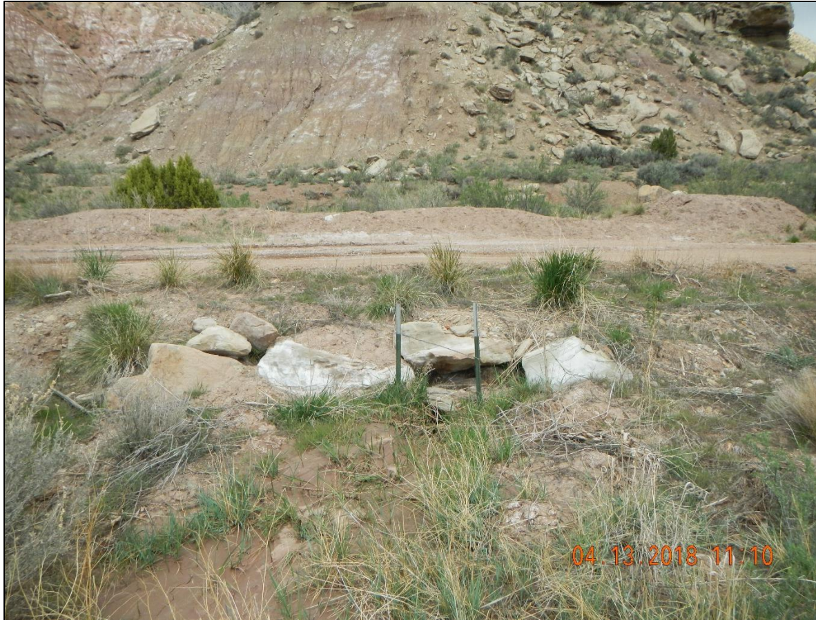
Sediment build up in culvert. 39.42103 108.08820
