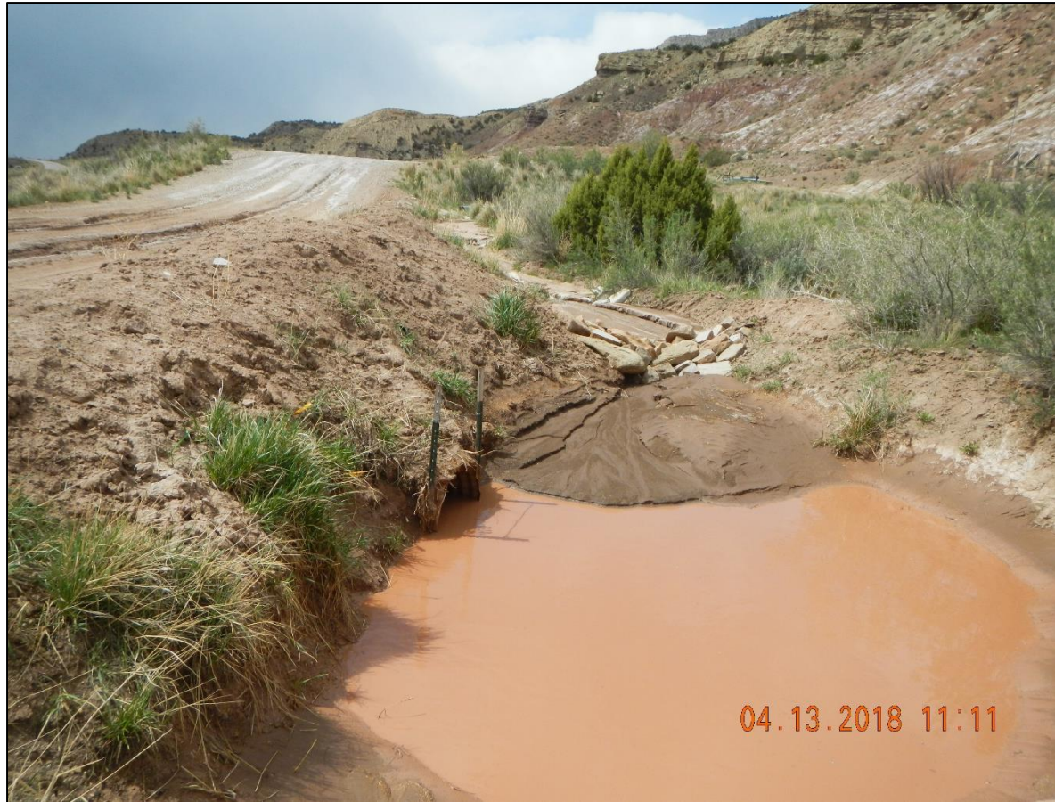
Sediment build up in culvert. 39.42103 108.08820
