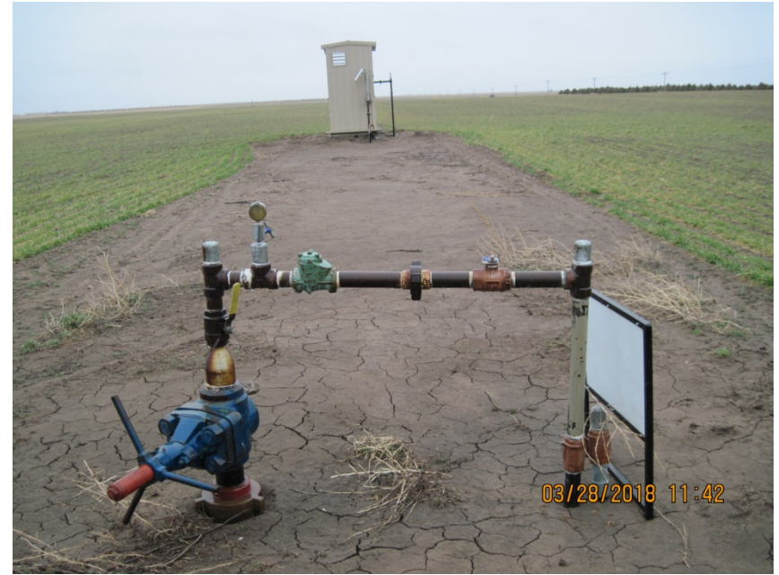
2. Meter shed & wellhead
