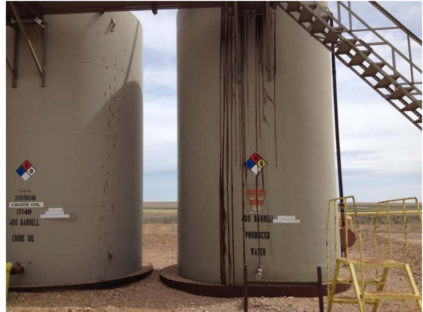
Photo 8 – produced water AST showing release from thief hatch.
