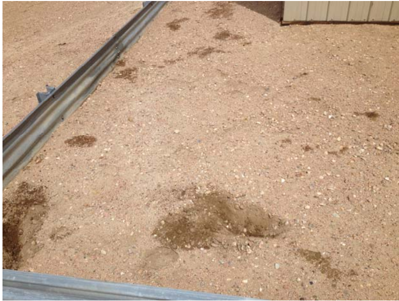
Photo 5 – Southwest corner of heater treater containment. Impacted soil within containment.
