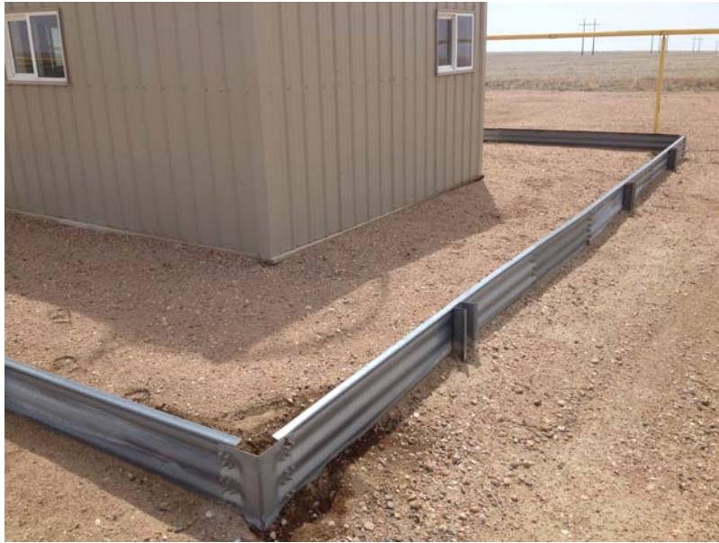
Photo 3 – Northwest corner of heater treater secondary containment. Impacted soil in foreground.
