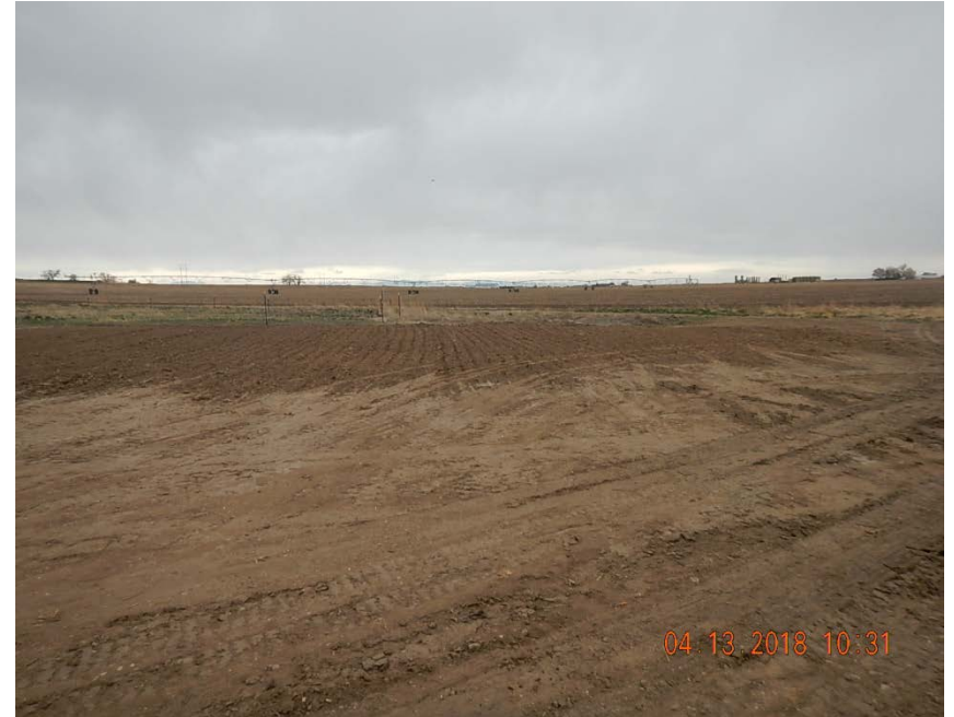
Photo 1: Meter run removed from battery location
