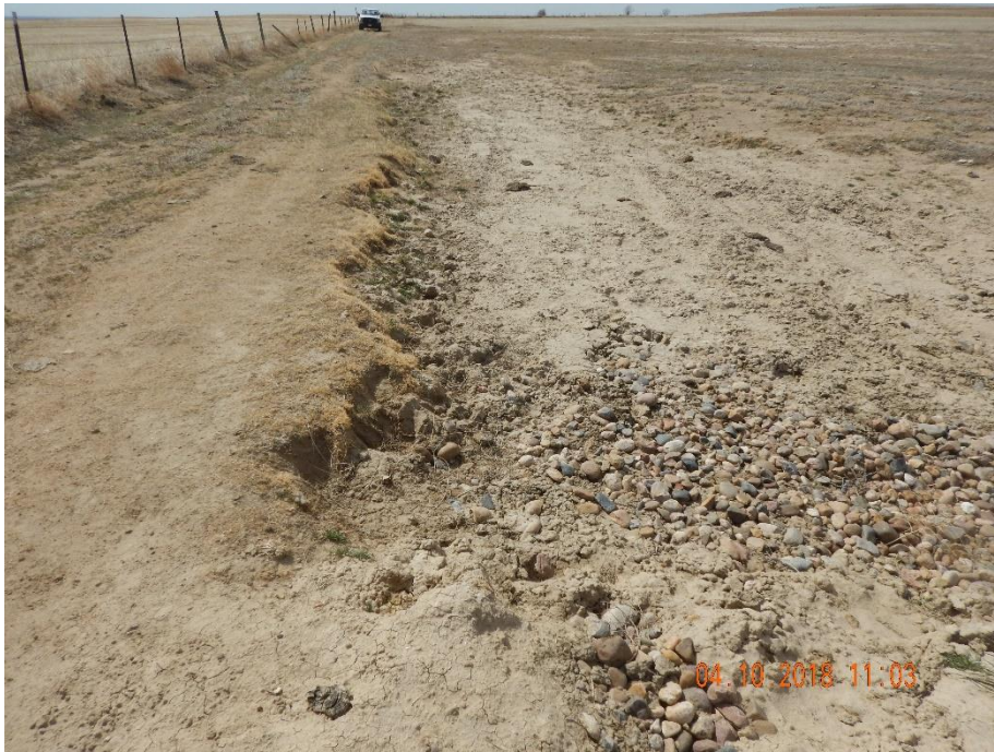
Photo 23: Photo taken from the southeastern end of the disturbance area, facing south. Photo shows stormwater erosion is beginning to once more degrade the location. Photos also shows no additional reclamation or remediation activities appear to have been conducted.
