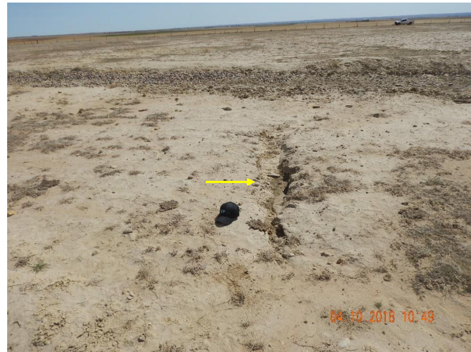
Photo 6: Photo taken from the southern end of the disturbance area, near the berm. Photo shows stormwater erosion is beginning to once more degrade the location. Active stormwater monitoring and management does not appear to be ongoing. Location does not appear to be sufficiently stabilized to prevent erosion degradation. Black ball cap for reference.
