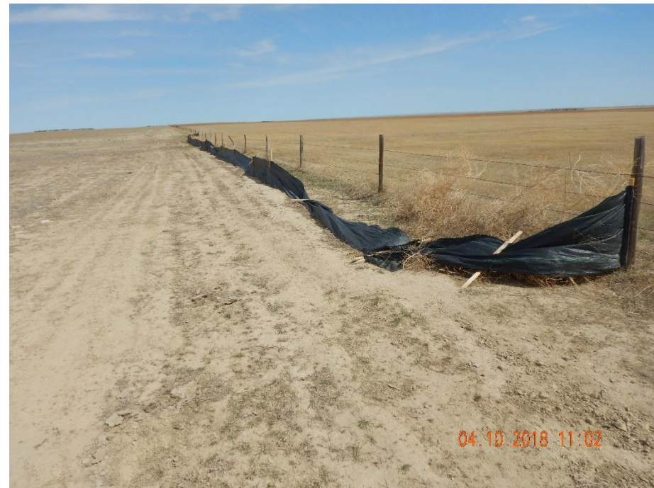
Photo 22: Photo taken from the northeast end of the disturbance area, facing north. Photo of silt fence BMP. Previous inspection documented that areas of the silt fence is already in disrepair and advised maintenance. Photo shows areas of the silt fence continues to be in disrepair.
