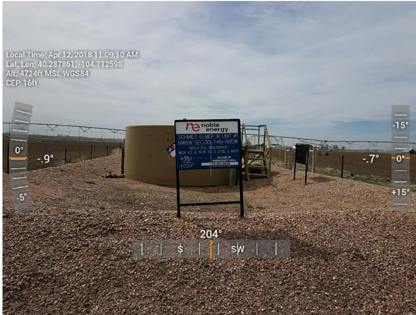
Tank battery signage
