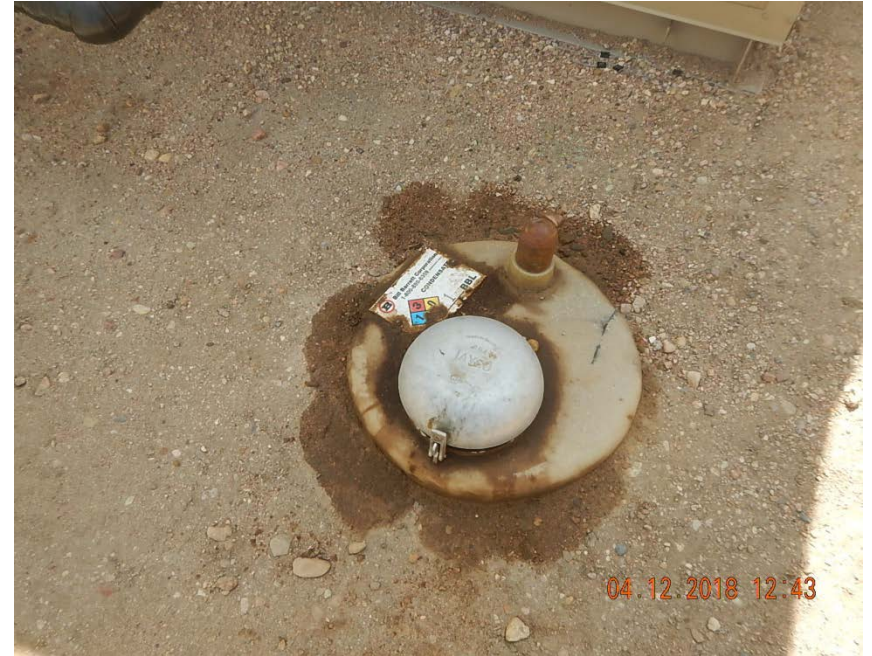
Photo 18: Stained soil at container at LACT.
