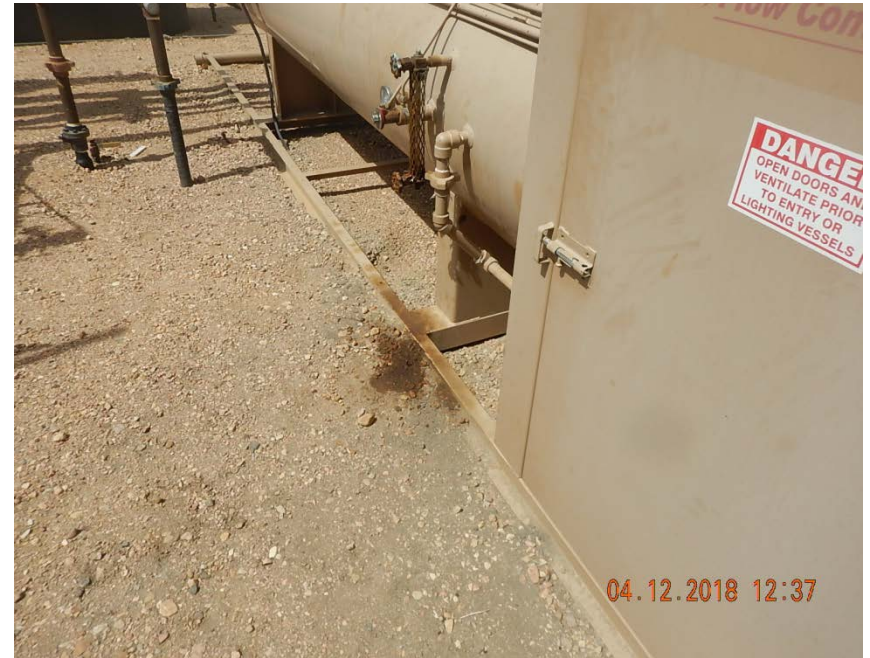
Photo 10: Stained soil near separator
