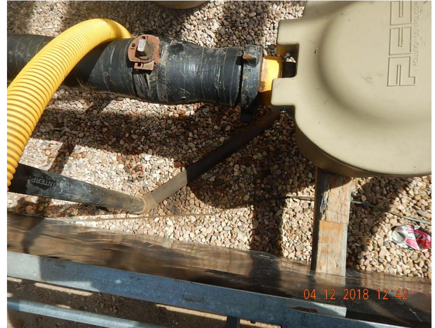
Photo 16: Stained soil at loadout.
