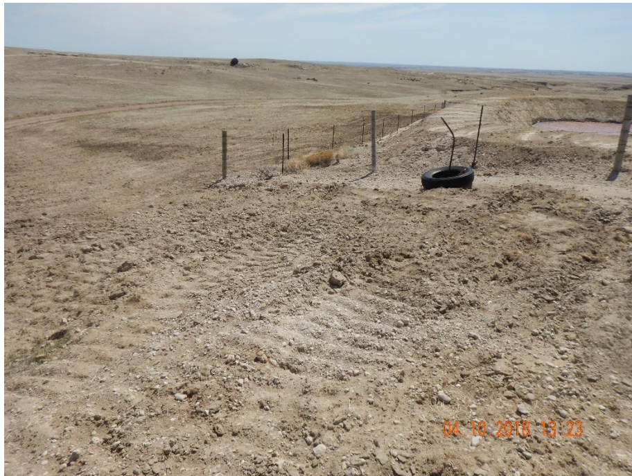
Photo 1: Photo taken from the east end of the location, facing southeast. Photo shows erosion degradation appears to have been repaired. However stabilization controls do not appear to have been implemented and revegetation activities do not appear to have been conducted.
