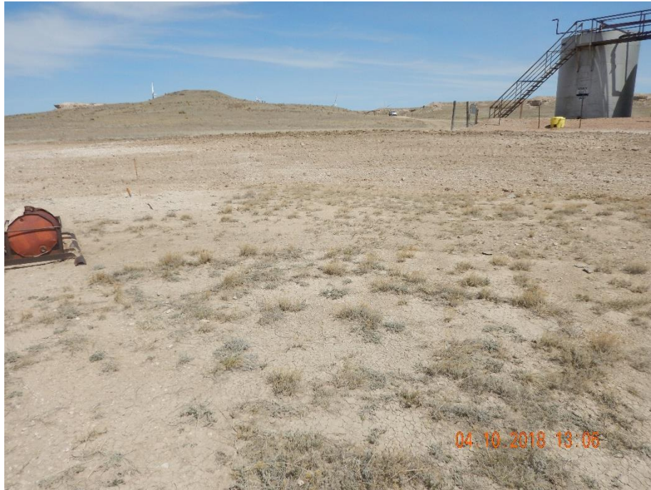
Photo 1: Photo taken from the central area of the location, facing north. Photo shows erosion degradation appears to have been repaired. However stabilization controls do not appear to have been implemented and revegetation activities do not appear to have been conducted.
