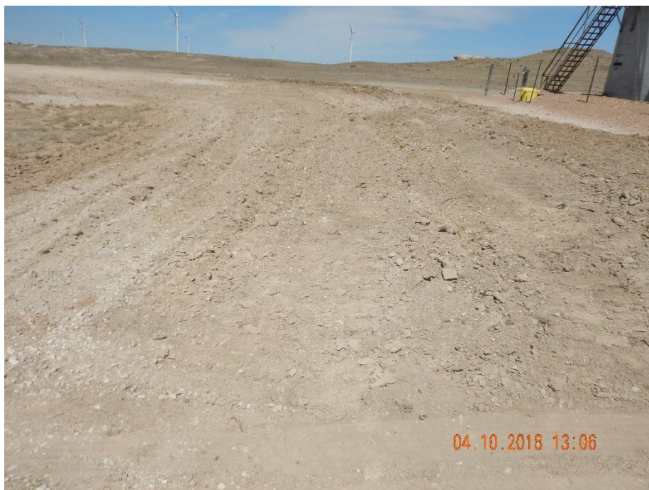
Photo 3: Photo taken from the central area of the location, facing east. Photo shows erosion degradation appears to have been repaired. However stabilization controls do not appear to have been implemented and revegetation activities do not appear to have been conducted.
