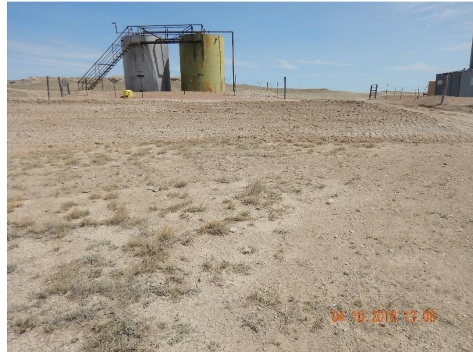
Photo 2: Photo taken from the central area of the location, facing east. Photo shows erosion degradation appears to have been repaired. However stabilization controls do not appear to have been implemented and revegetation activities do not appear to have been conducted.
