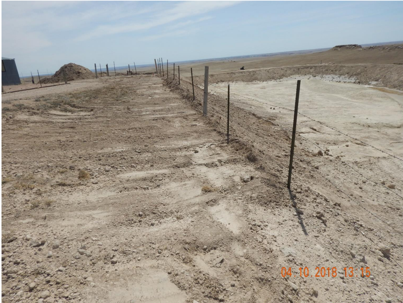
Photo 15: Photo taken from the east end of the pit. Photo shows gulley erosion has been repaired.
