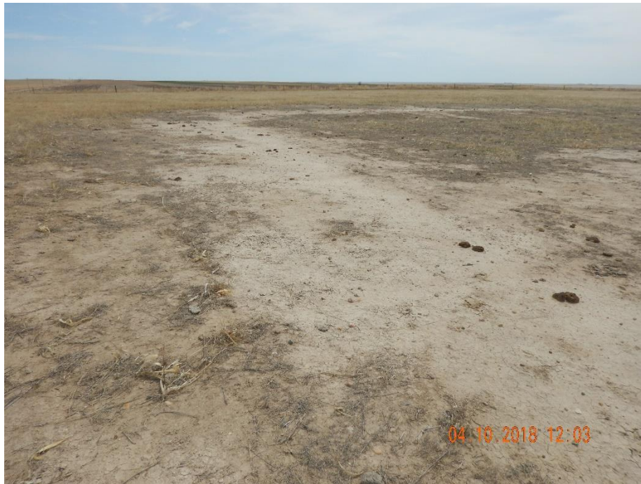
Photo 9: Photo taken from the northern end of the former pit locations, facing east. Photos 9-12 provide an overview of the pit locations from east to south to west. Photos show pit locations do not meet 1004.a reclamation requirements and standards. Area of the pits remains predominantly undesirable weedy plant species, or bare and exposed soil.
