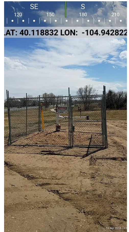
Photo 3 Pig Station Remaining at Former Battery Location
