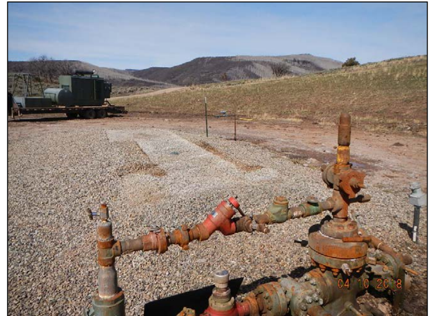
Photo 2. Pump jack had been removed. Equipment removal in process on location at the time of inspection.
