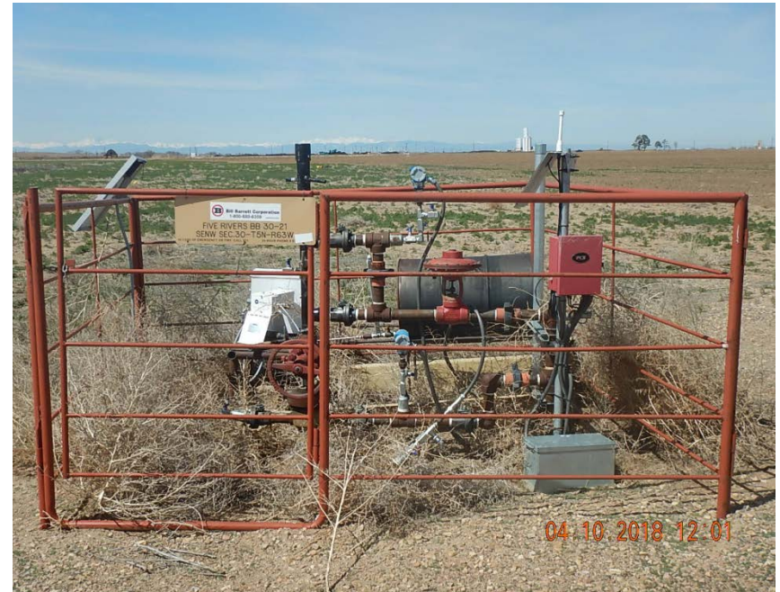
Photo 2: Wellhead, looking W
