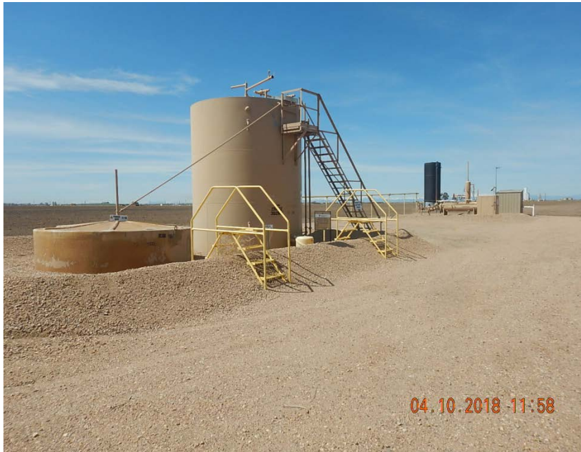
Photo 1: Location, looking SW
