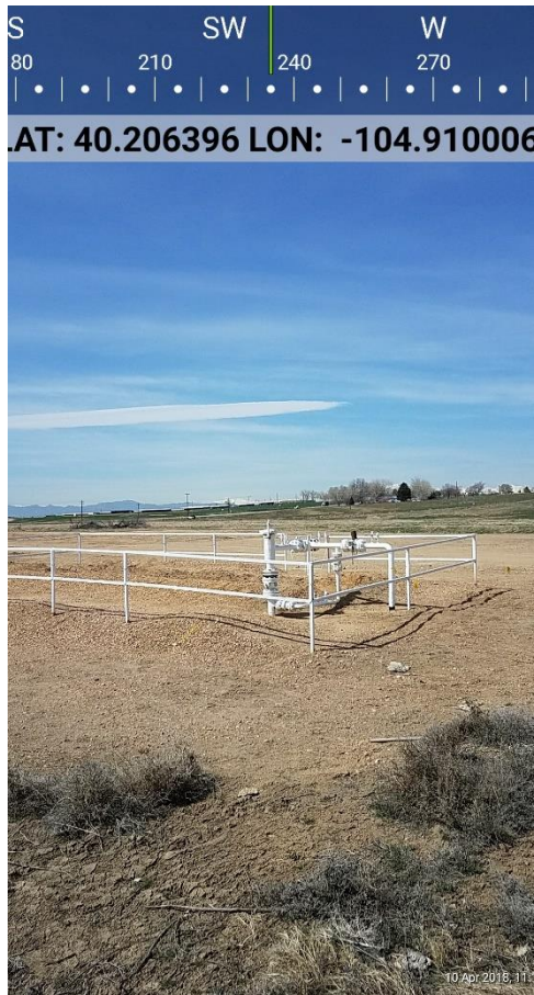
Photo 1 Location Overview from NE
