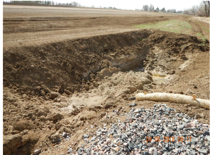
Photo 2. Photo taken from the northwestern well location on April 5, 2018, facing South. Appears the Operator built embankment berms and installed straw wattles, but did not stabilize the side slopes. Operator has encountered ground water which should not occur when installing a sediment trap.
