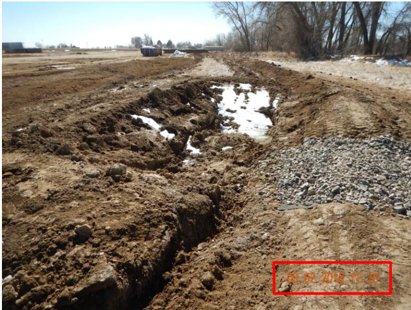
Photo 1. Photo taken from the northwestern well location on March 2, 2018, facing South. Operator has not installed the sediment trap in accordance with good engineering practices per Rule 1002.f.(2). Sediment trap side slopes are not stabilized, left unconsolidated. Sediment traps should not mix with ground water.
