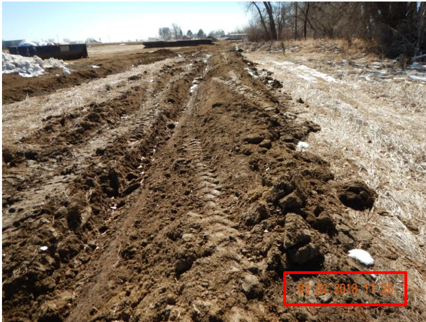
Photo 4. Photo taken from the western well location on March 2, 2018, facing South. The berm BMP along the western location has not been properly stabilized. An unconsolidated berm BMP is not a proper functioning BMP, as the unconsolidated material becomes a source of potential pollution itself. Perimeter of the well location is approximately 60 feet from the adjacent reservoir.
