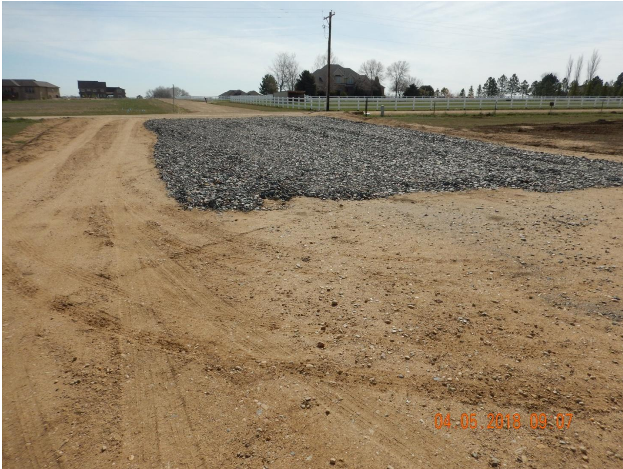
Photo 6. Photo taken from the entrance of the location on April 5, 2018, facing East. Appears the Operator has installed a tracking pad device along a portion of the location entrance. Appears there is a path along the tracking pad device with no BMPs.
