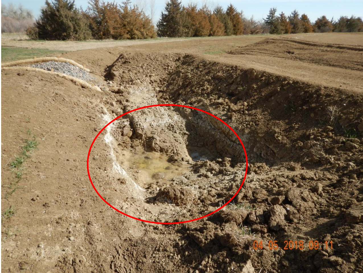
Photo 3. Photo taken from the northwestern well location on April 5, 2018, facing North. Photo illustrates unconsolidated side slopes and Operator has encountered ground water which should not occur when installing a sediment trap.
