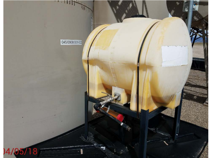
Missing signs on chemical container
