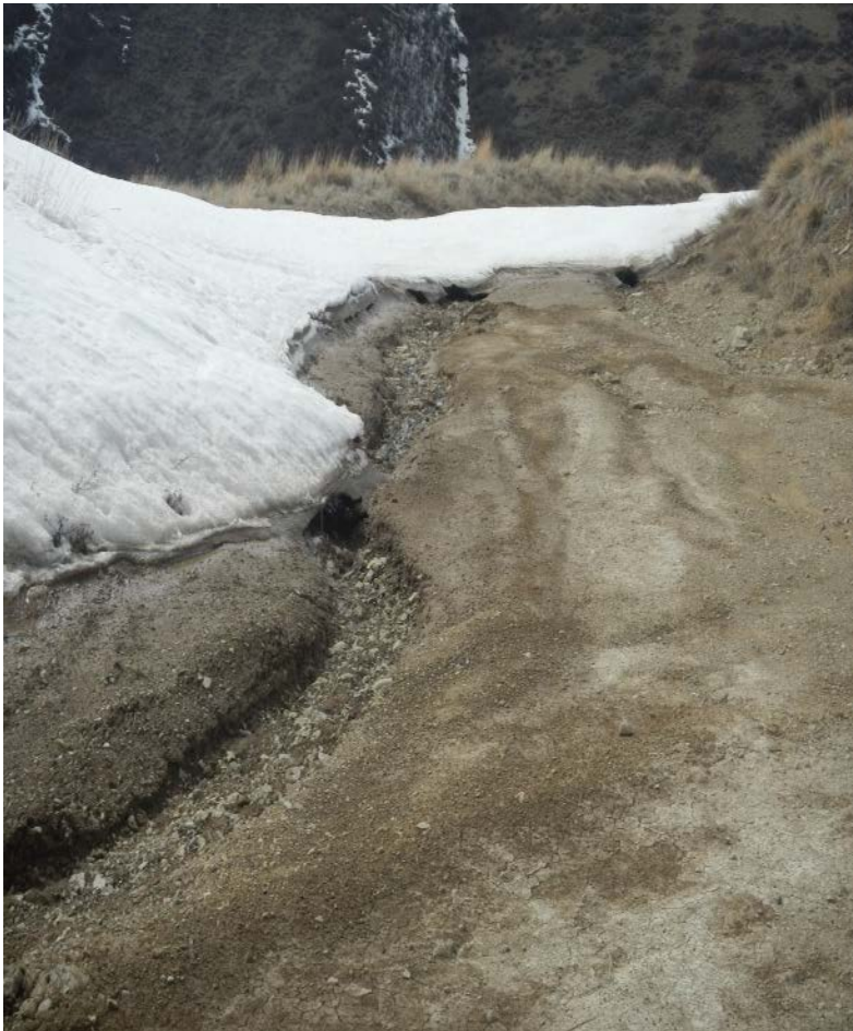
Photo#3: Erosion is occurring on road that leads off Southwest corner of pad.
