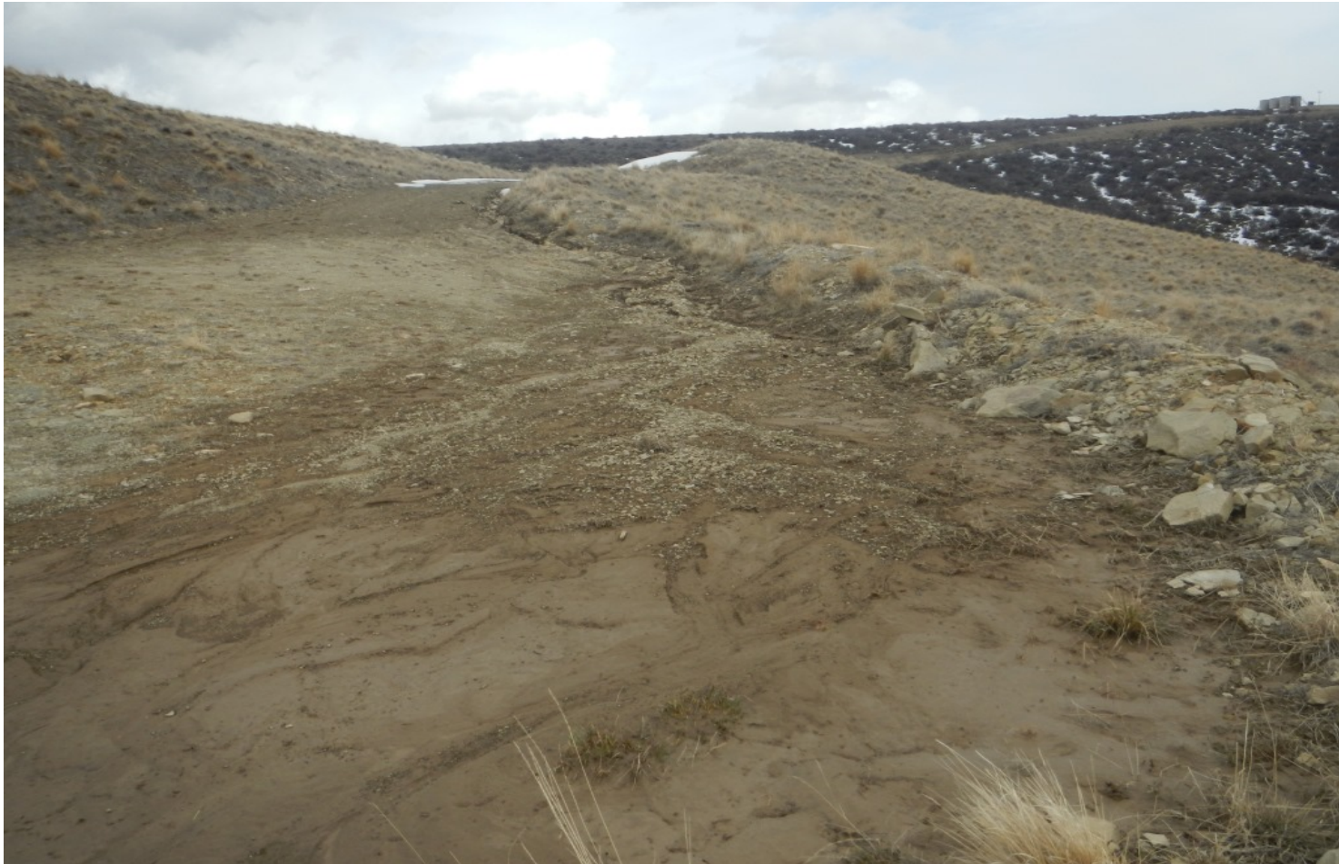
Photo#7: Sediment is being deposited at pooling area at end of road in previous photos.
