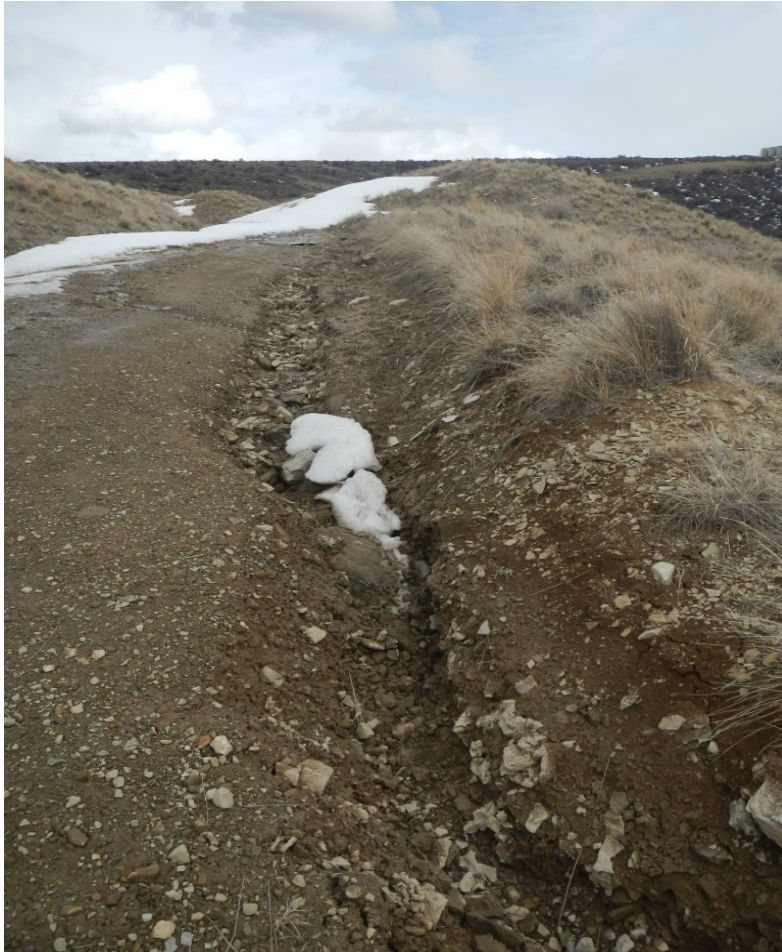
Photo#5: Erosion is occurring on road that leads off Southwest corner of pad
