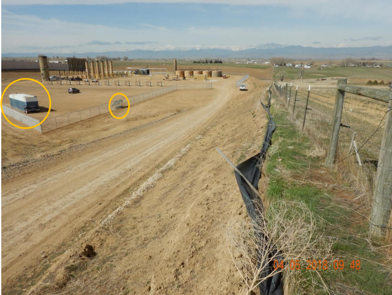
Photo 3. Photo taken from the entrance of the location, facing West. Operator has failed to maintain stormwater BMPs. Silt fence BMP in disrepair throughout the entire location. Also, there appeared to be other equipment stored along the eastern well pad location. Operator shall remove this equipment if it is not being used for production operations.
