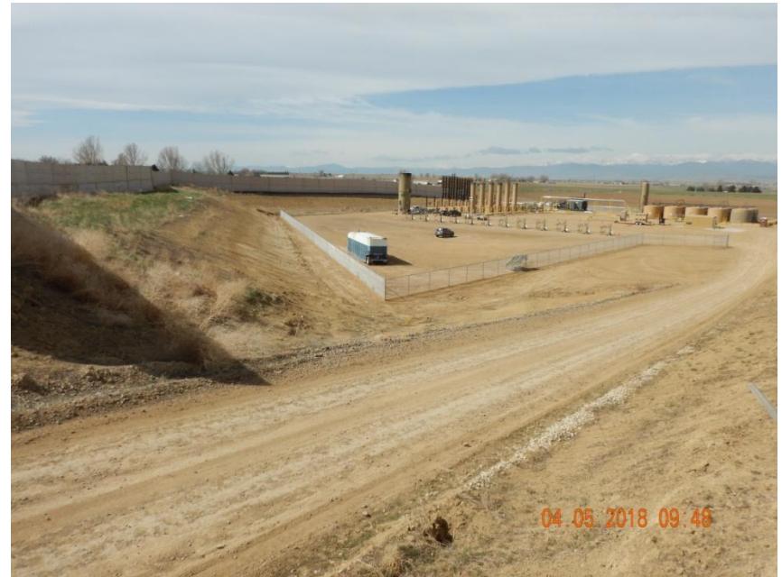
Photo 2. Photo taken from the entrance of the location, facing Southwest. Photo illustrates the Operator has failed to conduct interim reclamation on areas not needed for production operations. There a
