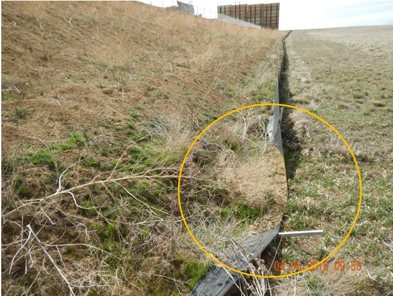
Photo 7. Photo taken from the discharge point along the northwestern location, facing South. Sediment discharge from gully erosion damaged the silt fence and discharged off location.
