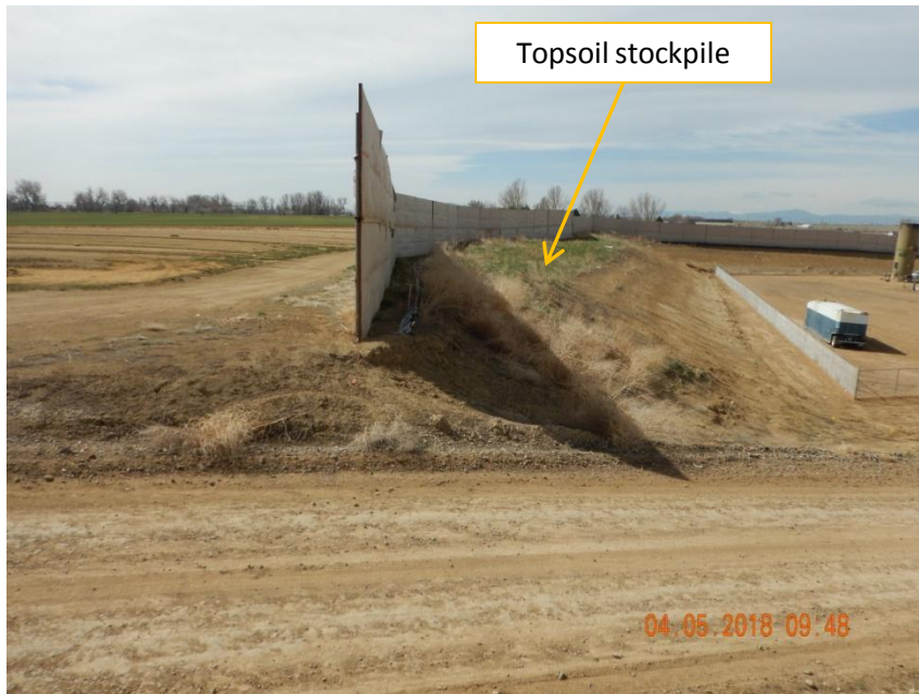
Photo 1. Photo taken from the entrance of the location, facing South. Appears topsoil was salvaged and stored along the eastern perimeter of the location. Note: Kochia weeds ( Kochia scoparia ) and weed debris were observed along portions of the location and was not managed and controlled. Kochia established on the fill slopes and topsoil stockpile.
