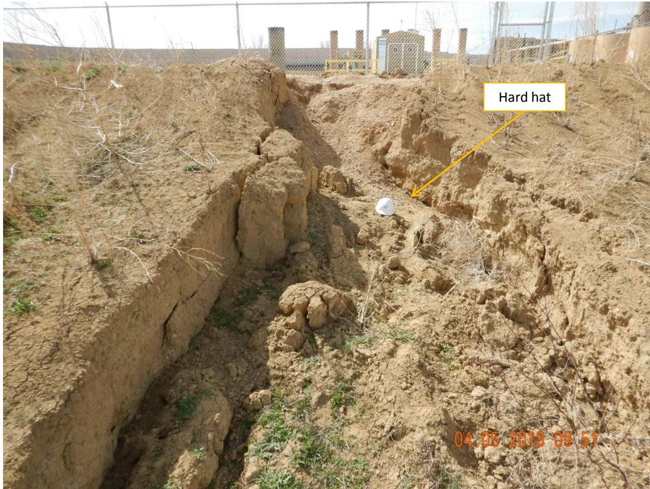
Photo 4. Photo taken from the northern location, facing South. Gully erosion up to three feet deep along the northern fill slopes. Sediment discharge off location was observed along the northwestern location- see Photo 7.
