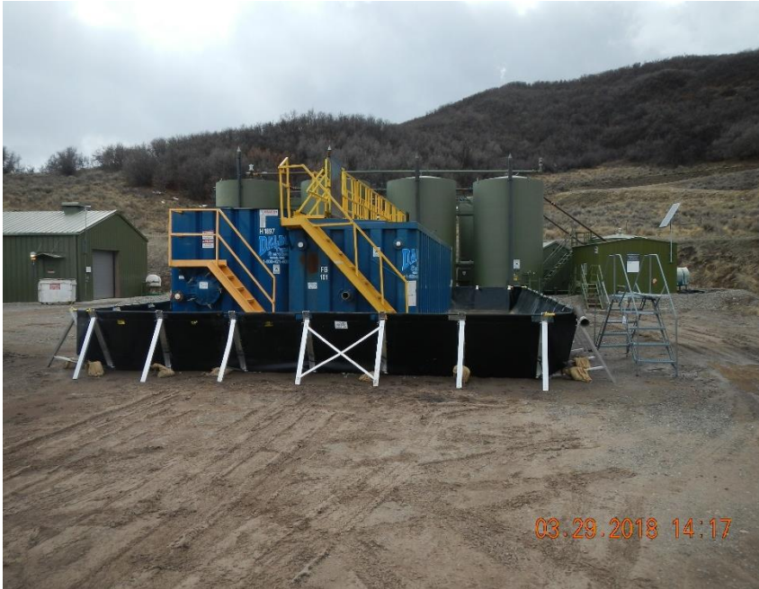
2 – 500 bbl. frac tanks labeled produced water in secondary containment.
