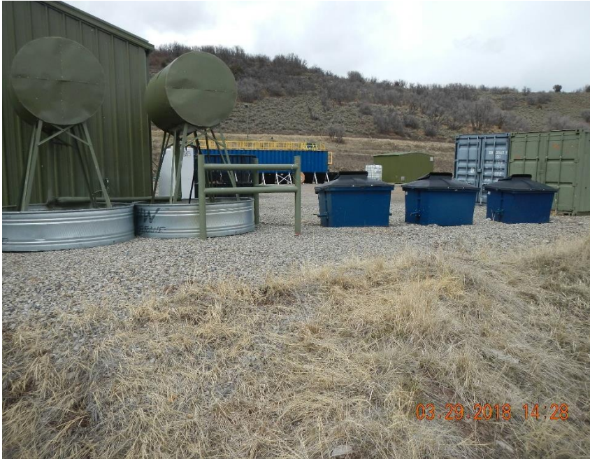
Rock drill and engine oil containers with secondary containment.
