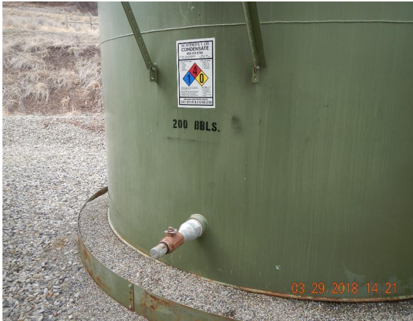
200 bbl. tank also labeled condensate.
