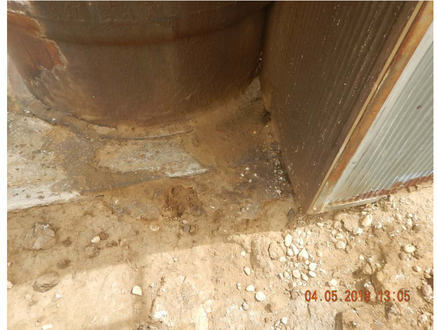
Photo 9: Stained soil at vessel
