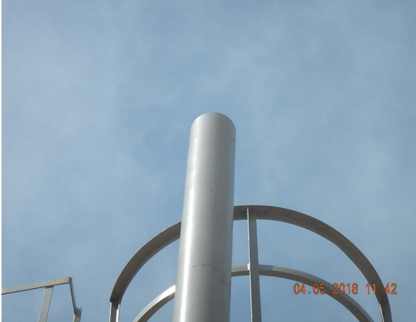
Photo 12: No screen on stack
