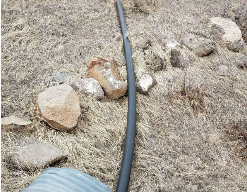
Pipe in or near culvert
