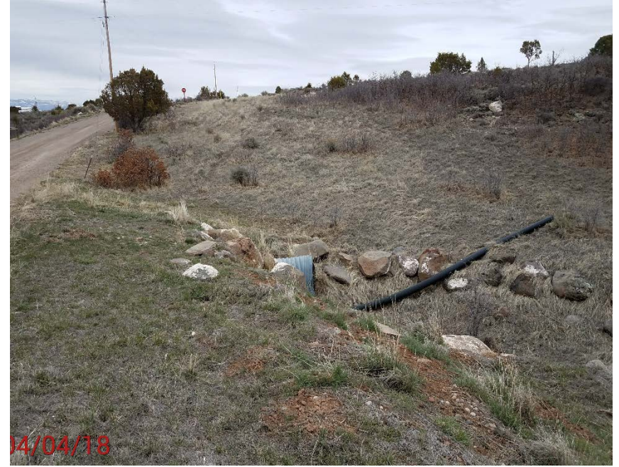
Pipe near culvert
