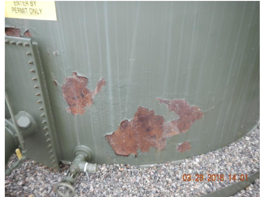
Peeling paint and rust present on second AST.
