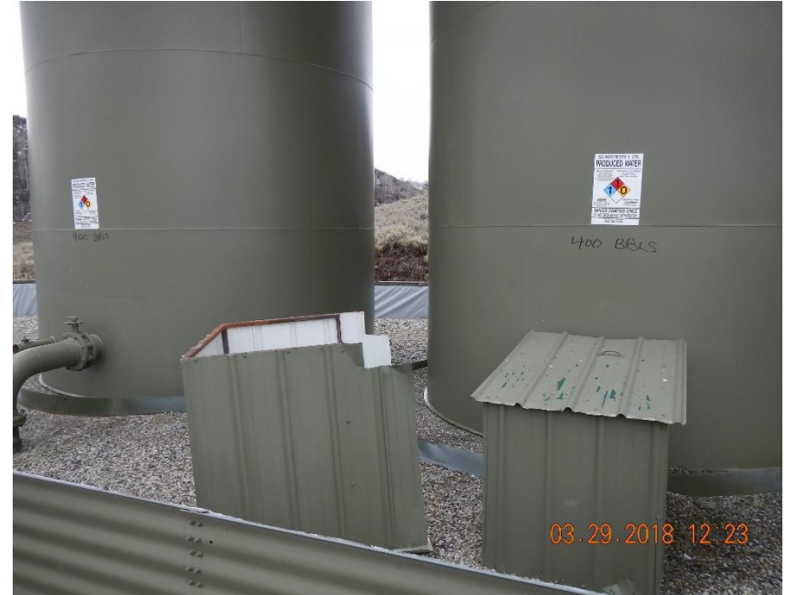
ASTs have NFPA placards and are labeled with contents and capacity.
