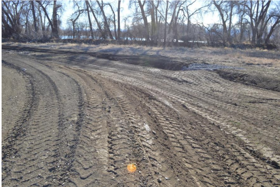
Photo 5. Photo showing stabilization of sediment trap on NW corner of location. (3/16/18)
