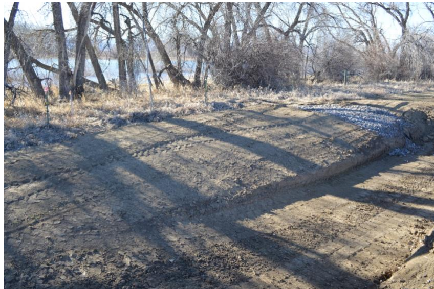
Photo 2. Photo showing stabilization of the sediment trap on the SW corner of the pad. (3/16/18)
