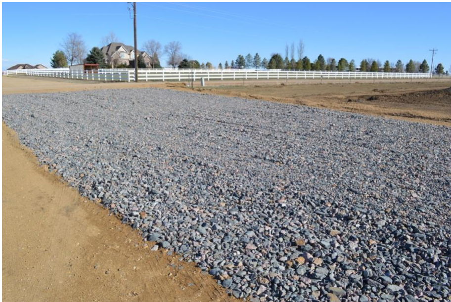
Photo 6. Photo looking SE showing vehicle tracking pad installed at entrance. (3/16/18)
