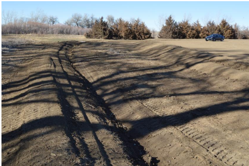
Photo 4. Photo looking north showing compaction of berm on west side of location. (3/16/18)
