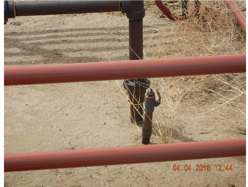
Photo 4: Riser at wellhead, plugged
