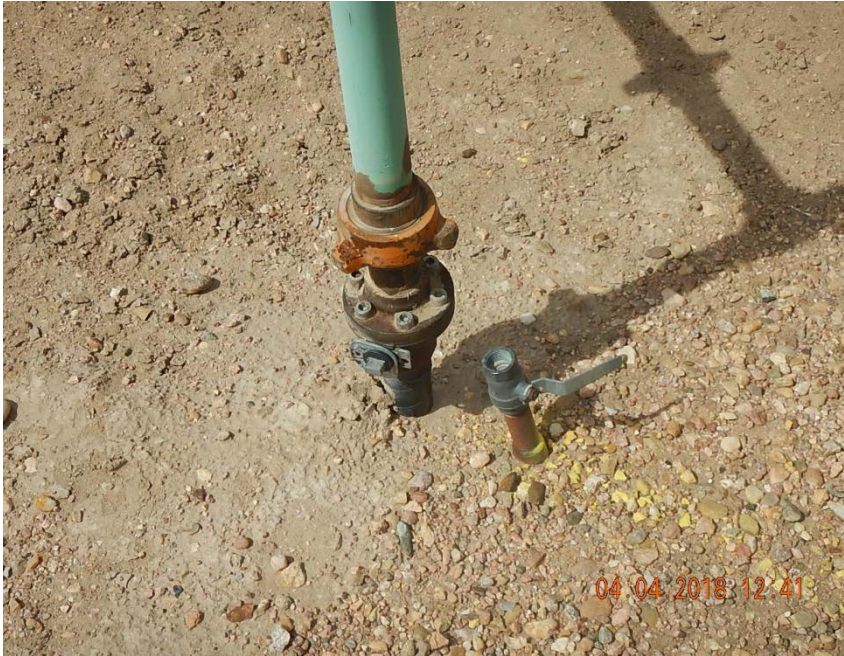
Photo 3: Riser not LO/TO at separator
