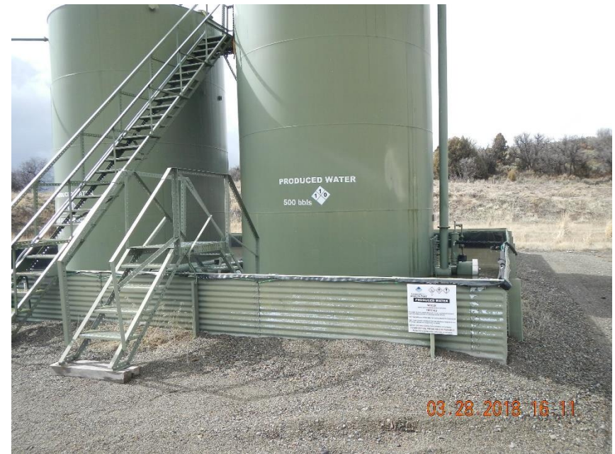
2 – 500 bbl. produced water heated ASTs.
