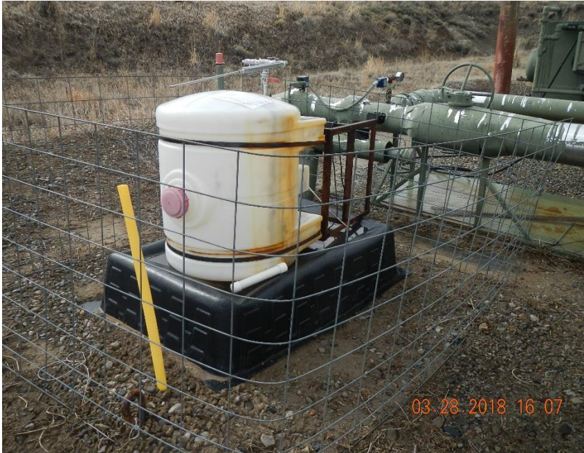
Unused chemical injection system.
