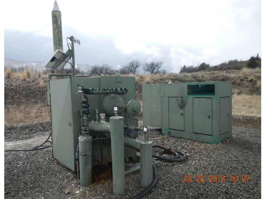
Horizontal heated separator and generator.
