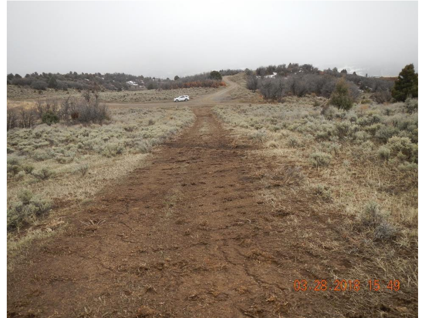
Water bars and slope roughening controlling erosion along access.
