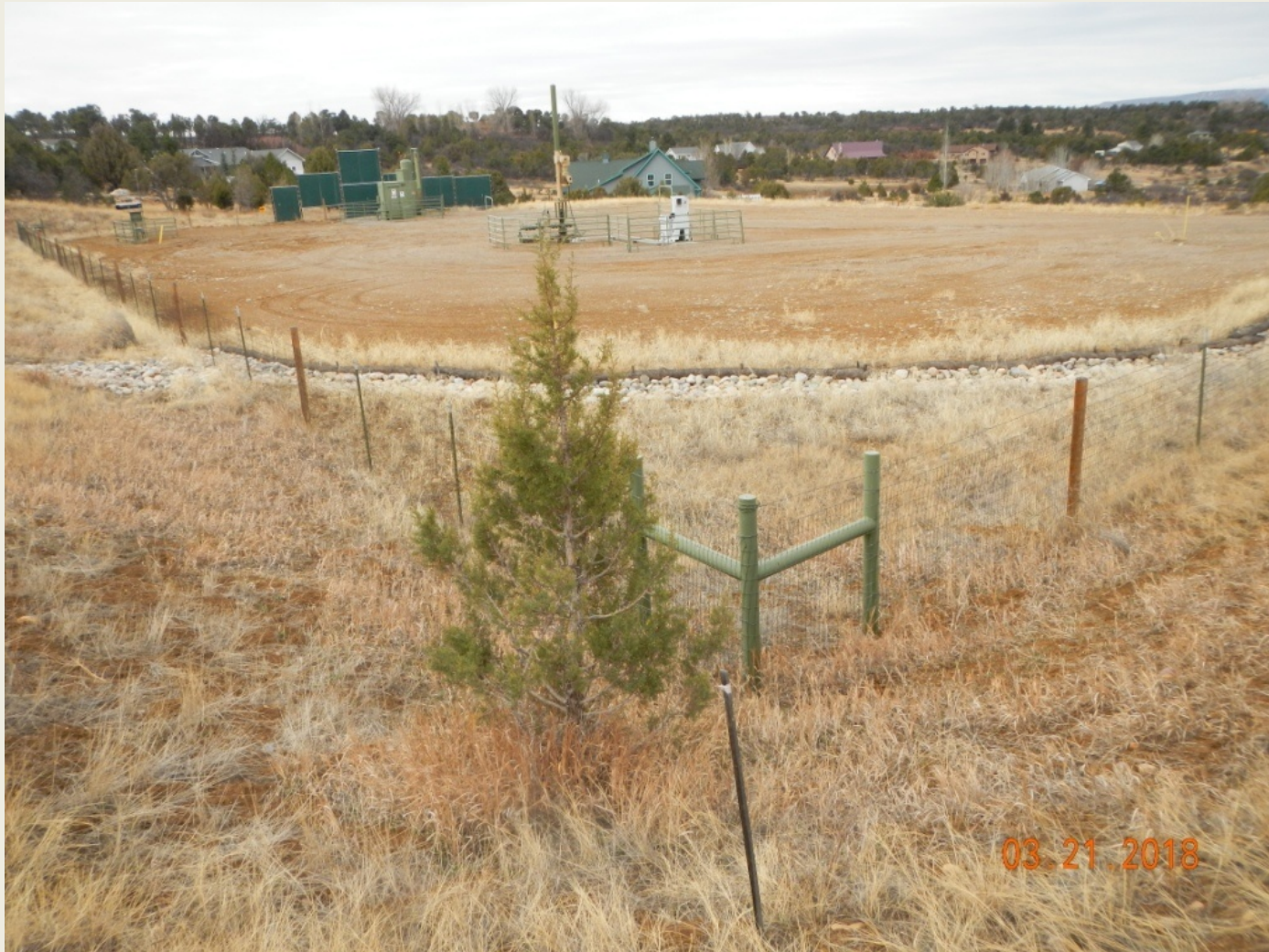
Photo 1. View of the project area from the northeastern corner facing center. Erosion controls are in place and appear to be functioning.
