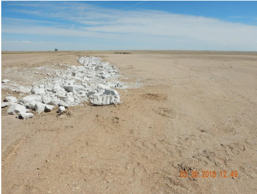
Photo 1. Photo taken from the northwest perimeter of the location, facing East. Waste on location from recent drilling operations needs to be removed per Rule 603.f.
