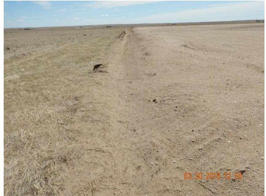
Photo 2. Photo taken from the northeast perimeter of the location, facing South. Appears to be a ditch installed along the eastern perimeter of the location. This was the only observed stormwater BMP, other than gravel at the location.
