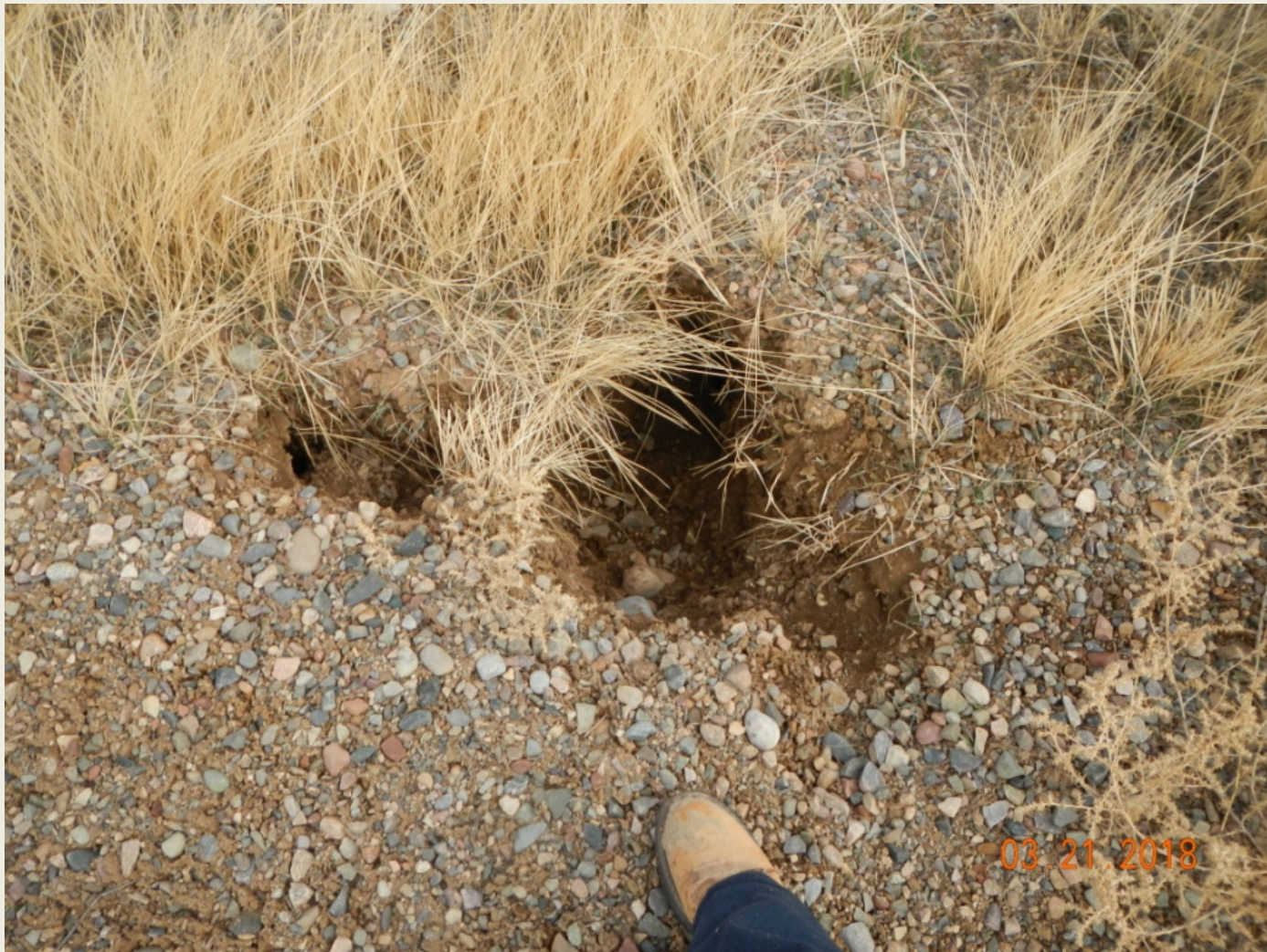
Photo 4. View of erosional tunneling that is starting to occur within the northern fill slope.
