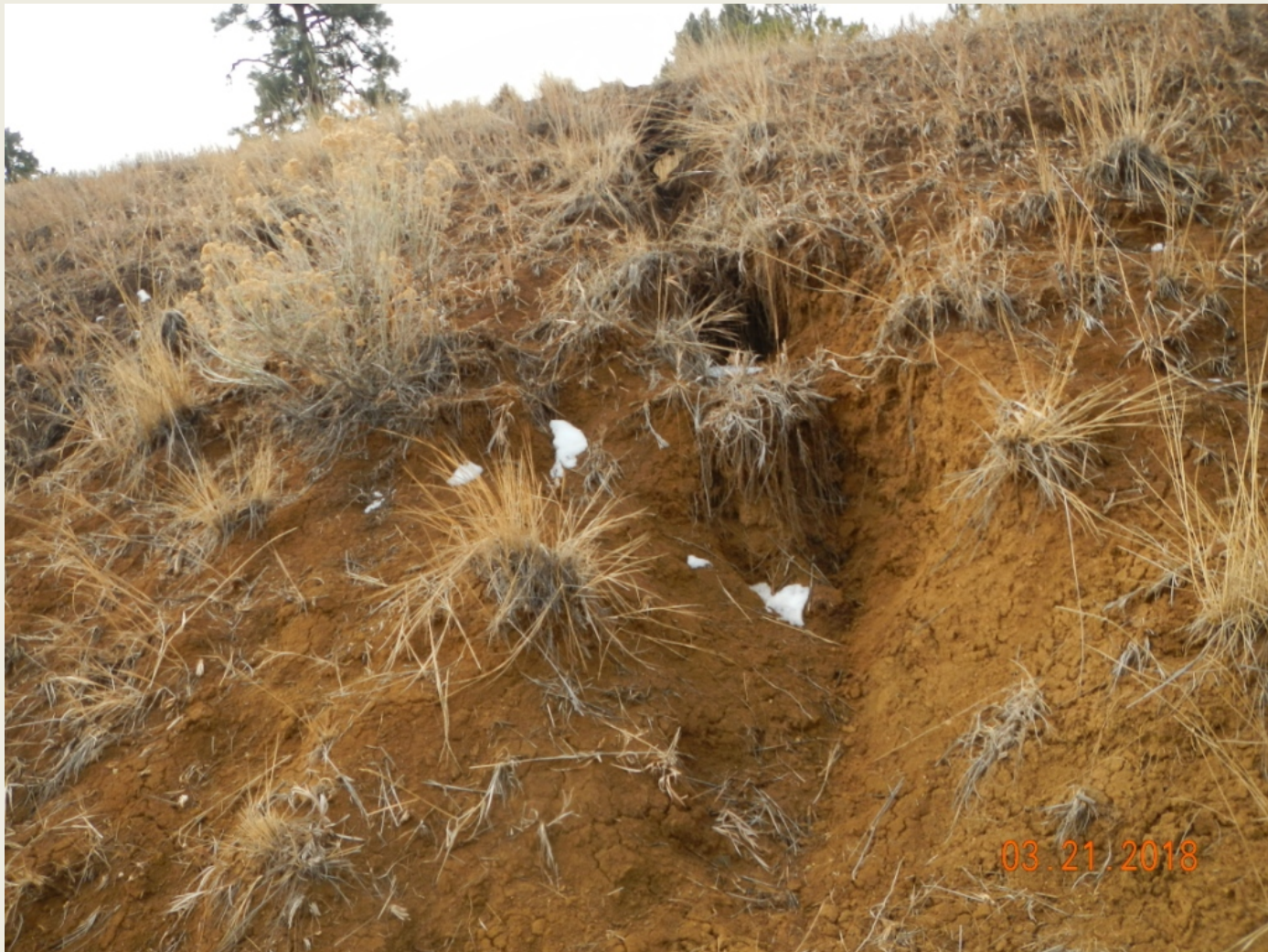
Photo 5. View of erosional channeling in the southern cut-slope Stabilization measures are needed here.
