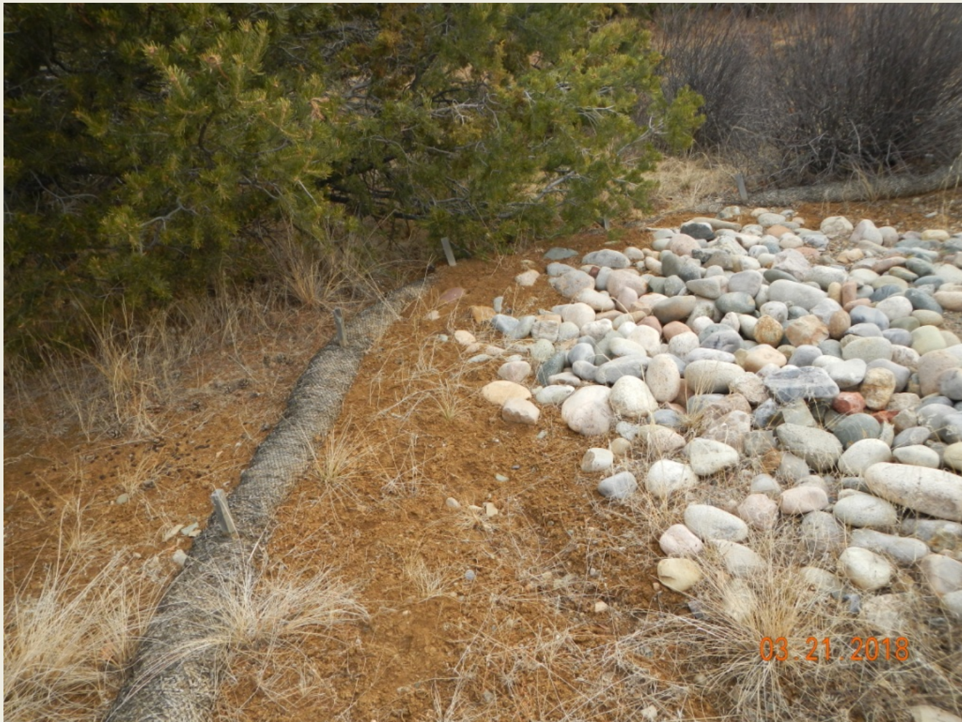
Photo 6. View of stormwater controls in the northeastern portion of the project area, that are filling with sediment and need maintenance.
