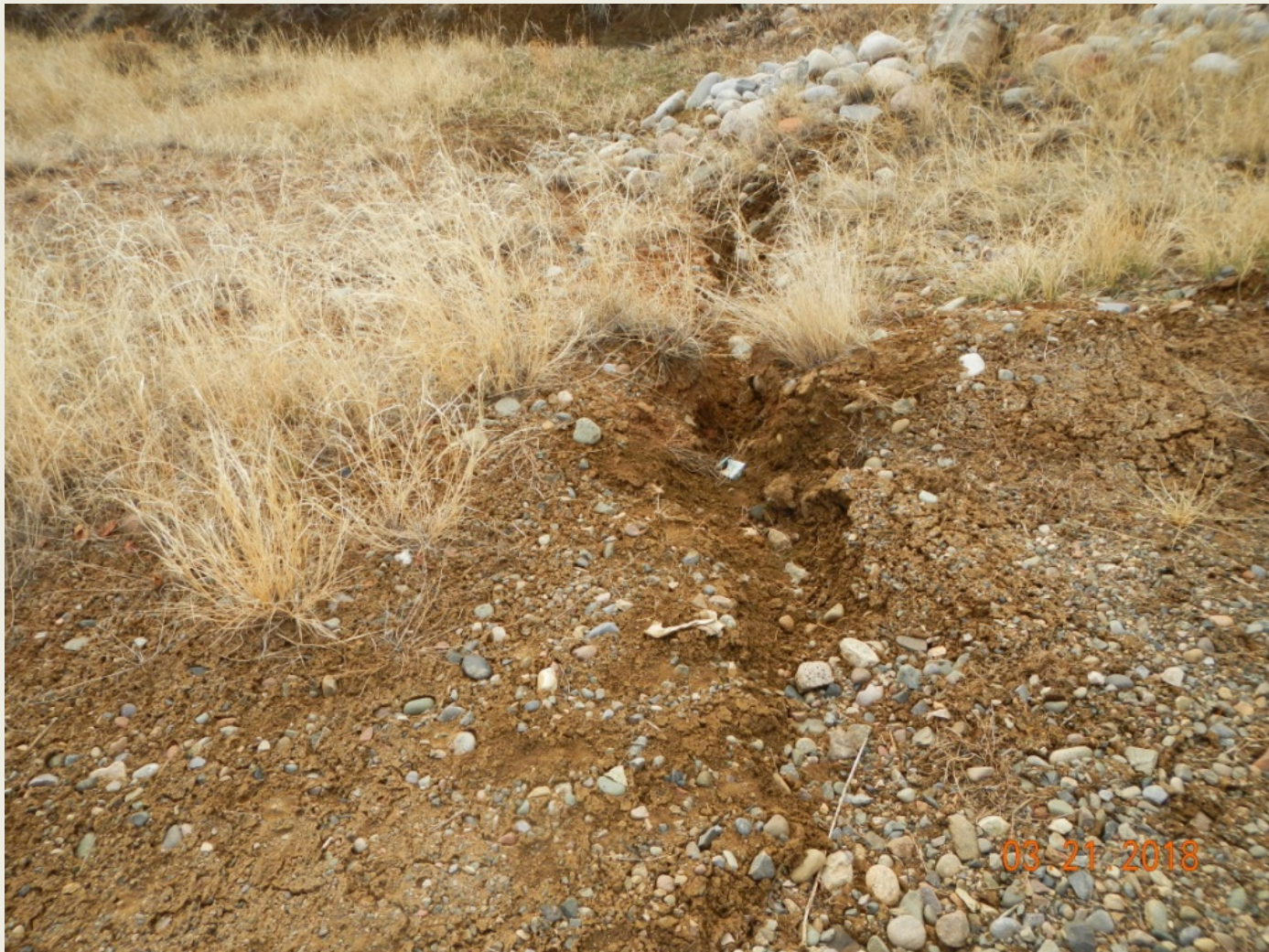
Photo 5. View of erosion occurring along the eastern edge of the well pad where stormwater flows from the well pad into a drainage. Stormwater controls are placed here, but additional stabilization is needed.
