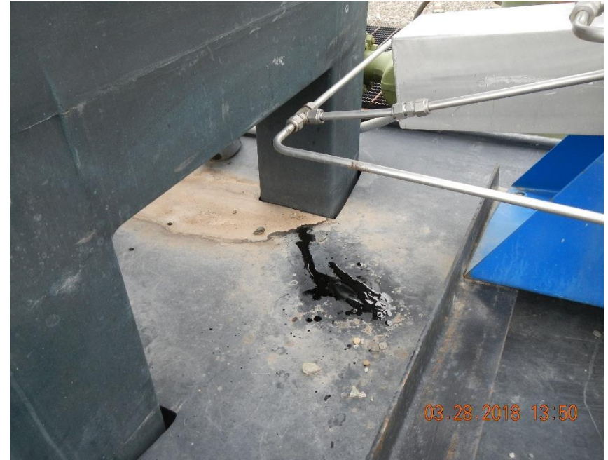
Stainless tubing on chemical injection system at DGU Hotchkiss Federal 1289 #18-H1 leak.
