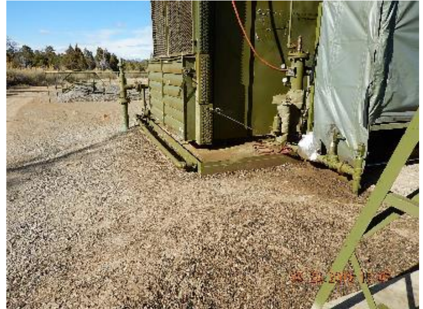
Photo 6: Closer view of impacted soil and gravel on S and SW side of compressor unit.
