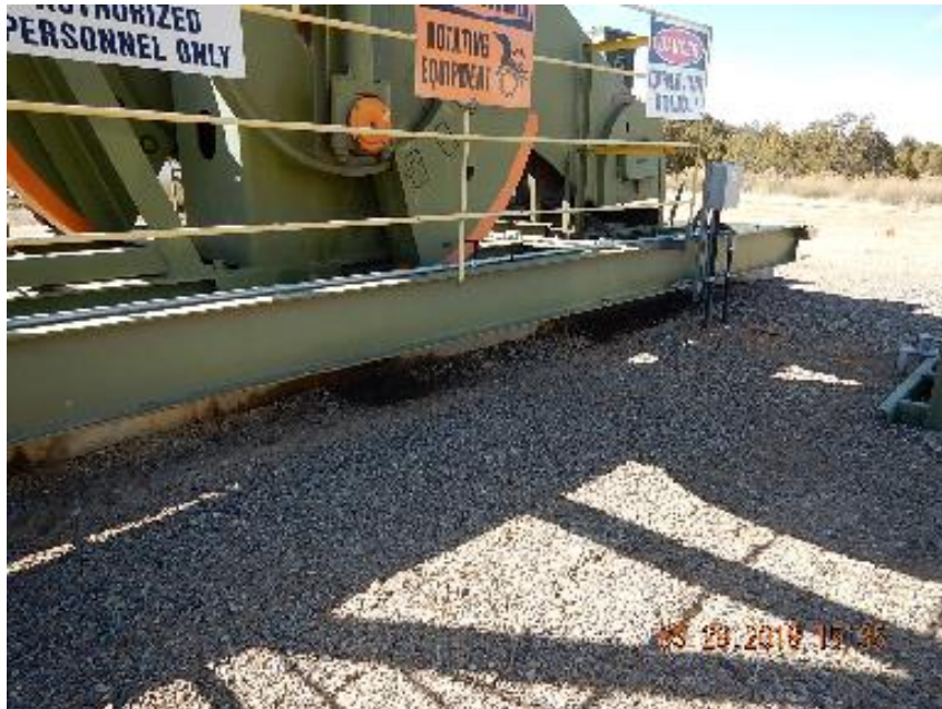
Photo 3: Impacted soil and gravel along concrete base of pump jack.
