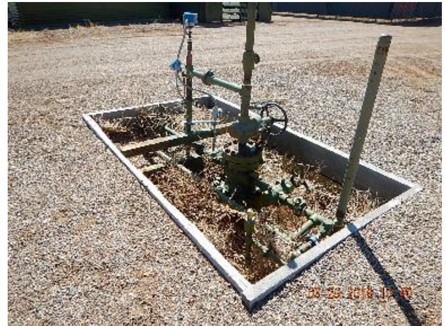
Photo 2: Debris blown into wellhead cellar.
