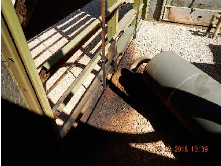
Photo 3: Impacted soil and gravel at compressor exhaust muffler.
