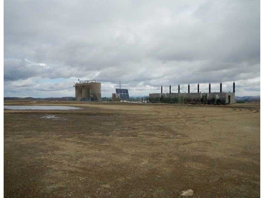
Location showing ASTs and separators
