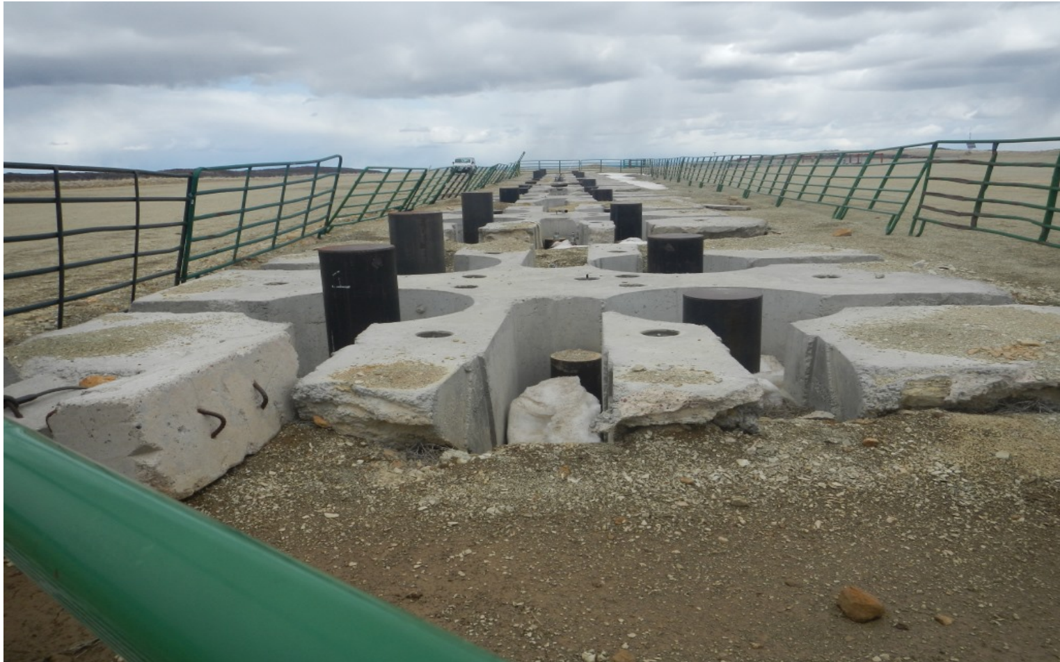
Photo#4: View over thirty –two Conductors set.
