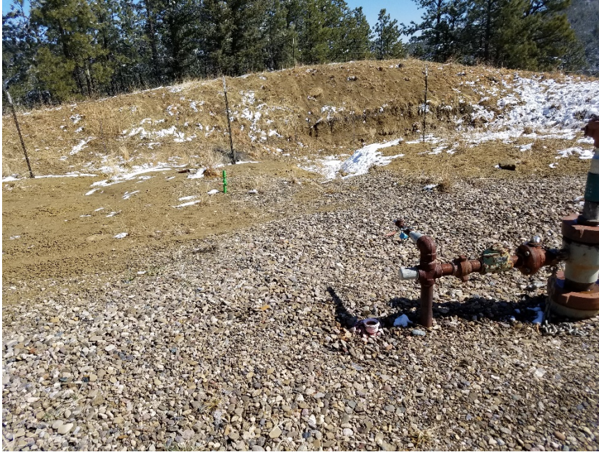
Photo 3. 2 unmarked risers
