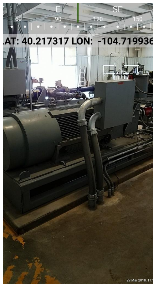
Photo 7 500HP Electric powered pump serving API 05-123-29168
