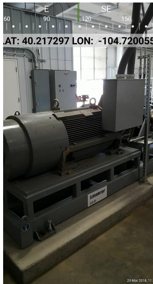
Photo 8 450HP Electric powered pump serving API 05-123-14349
