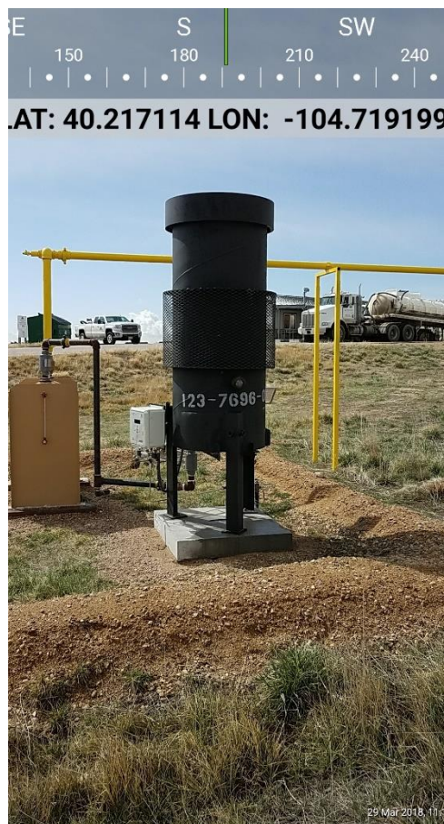
Photo 10 Emission Control Burner
