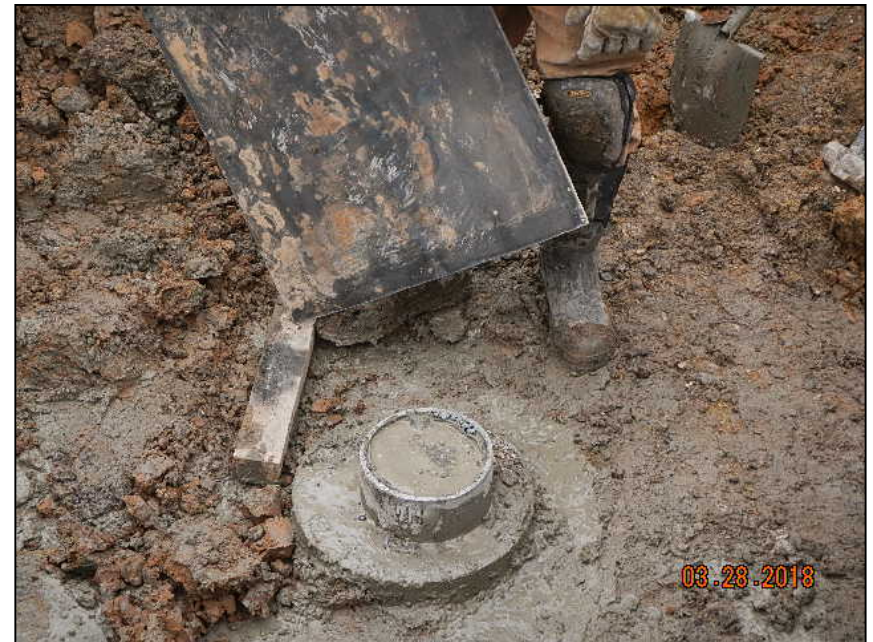
Photo 2. Cement to surface.
