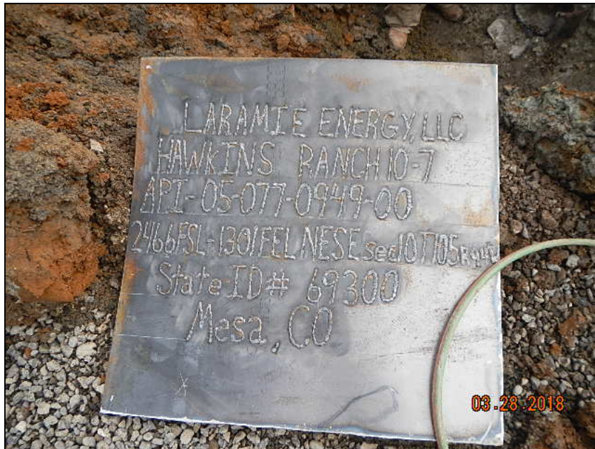
Photo 1. Plate for PA Well.
