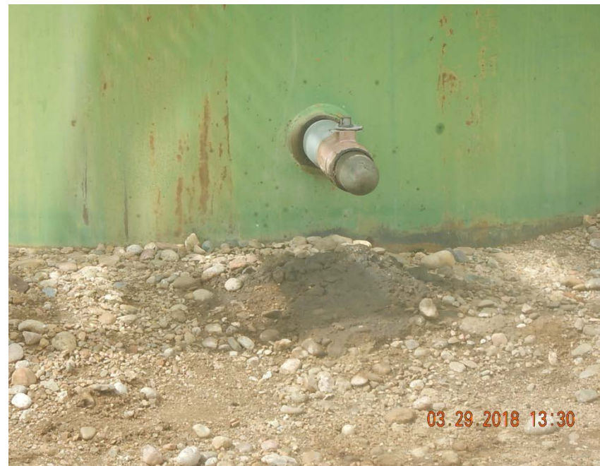
Photo 20: Stained soil at crude oil loadout.
