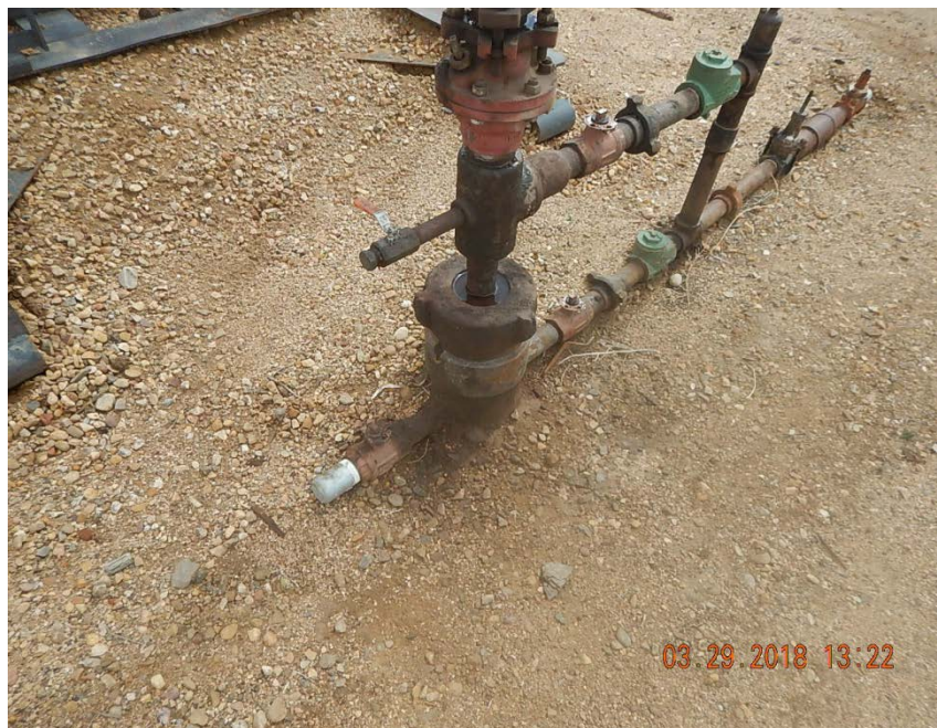
Photo 5: Stained soil at Dacono 3 wellhead
