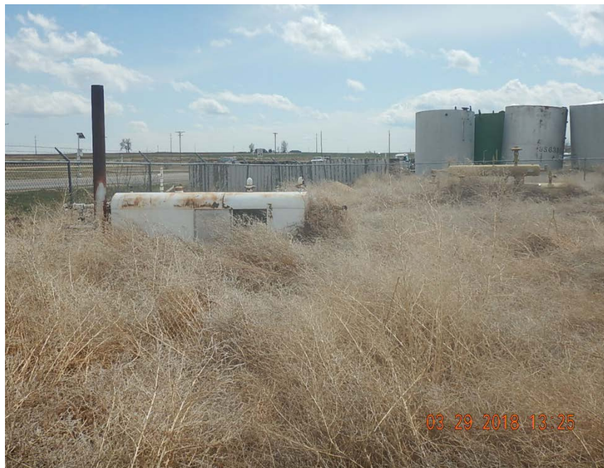
Photo 11: Unused horizontal separators on SE corner of location
