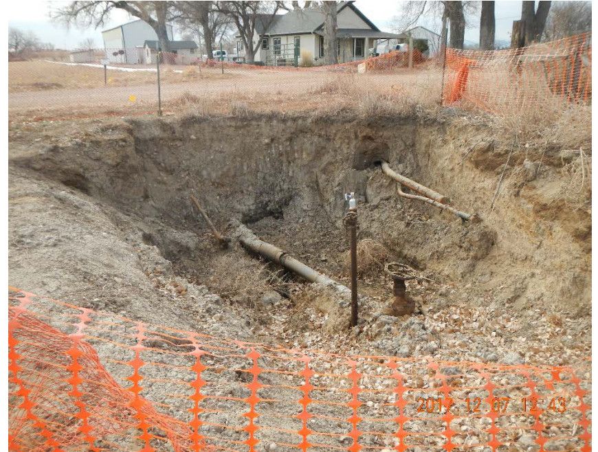
Piping visible in excavation
