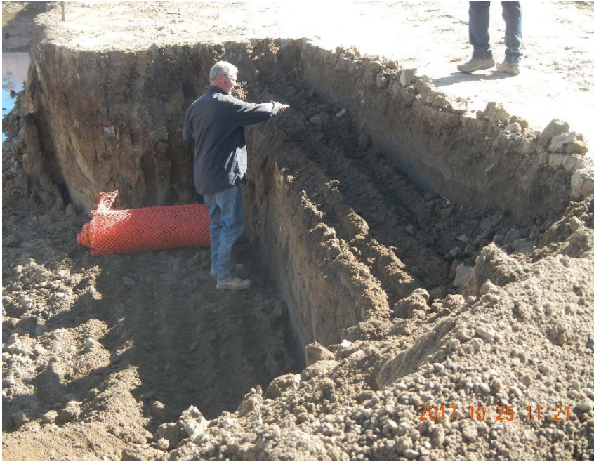
Field Screening walls of the excavation
