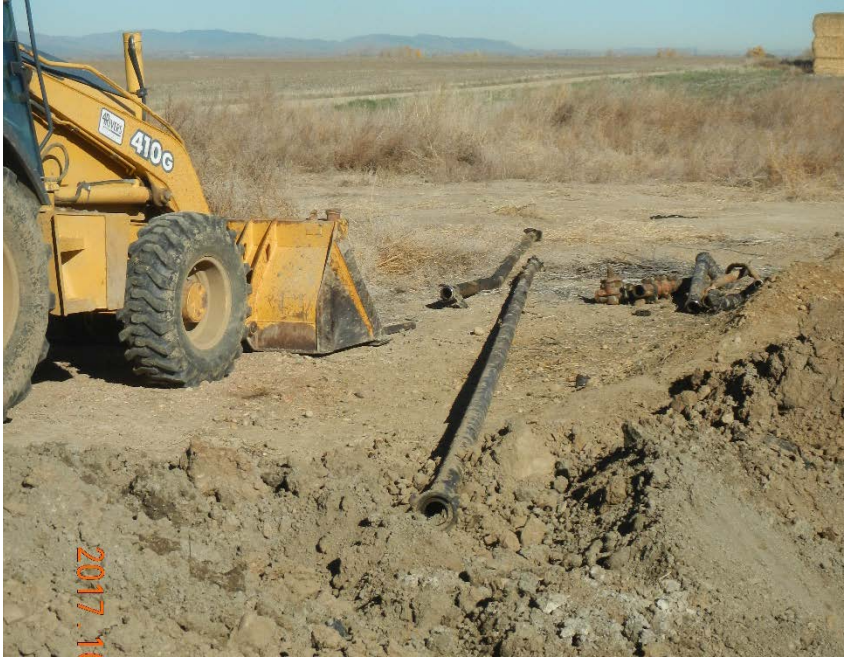
Piping remove from excavation
