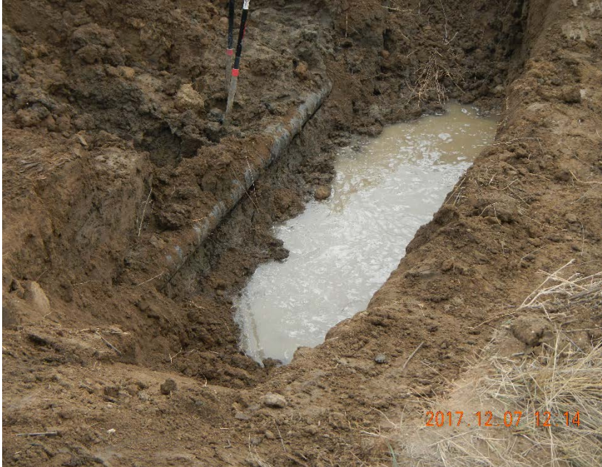
Ground water entering open excavation
