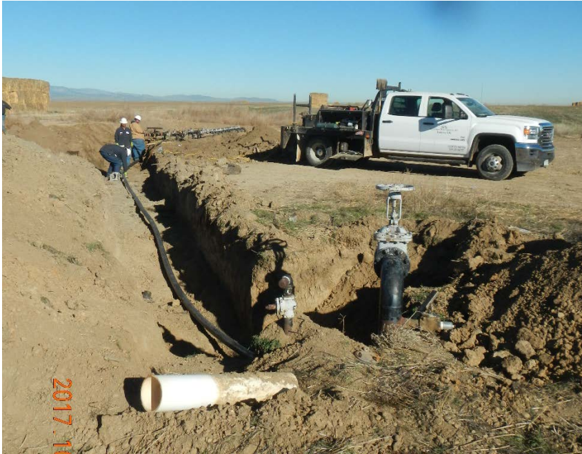
Flowline repairs
