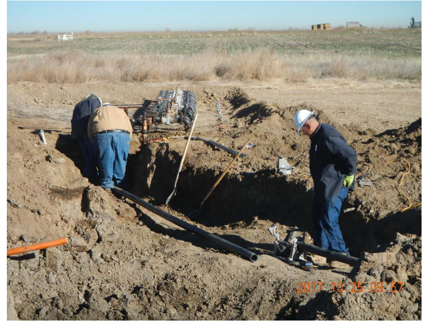
Flowline repairs
