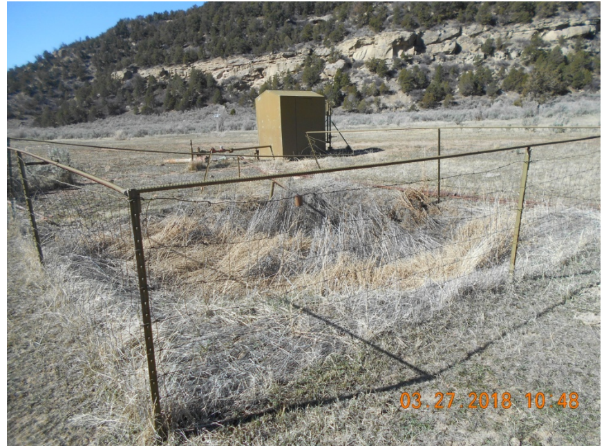
Blowdown pit with fencing.
