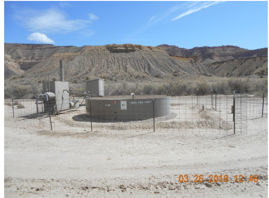
Separator, Meter housing and tank with fencing
